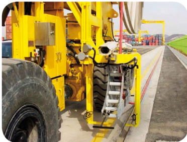
Video cameras monitor the cable trench to assure that the cable remains free to pay out and wind up
